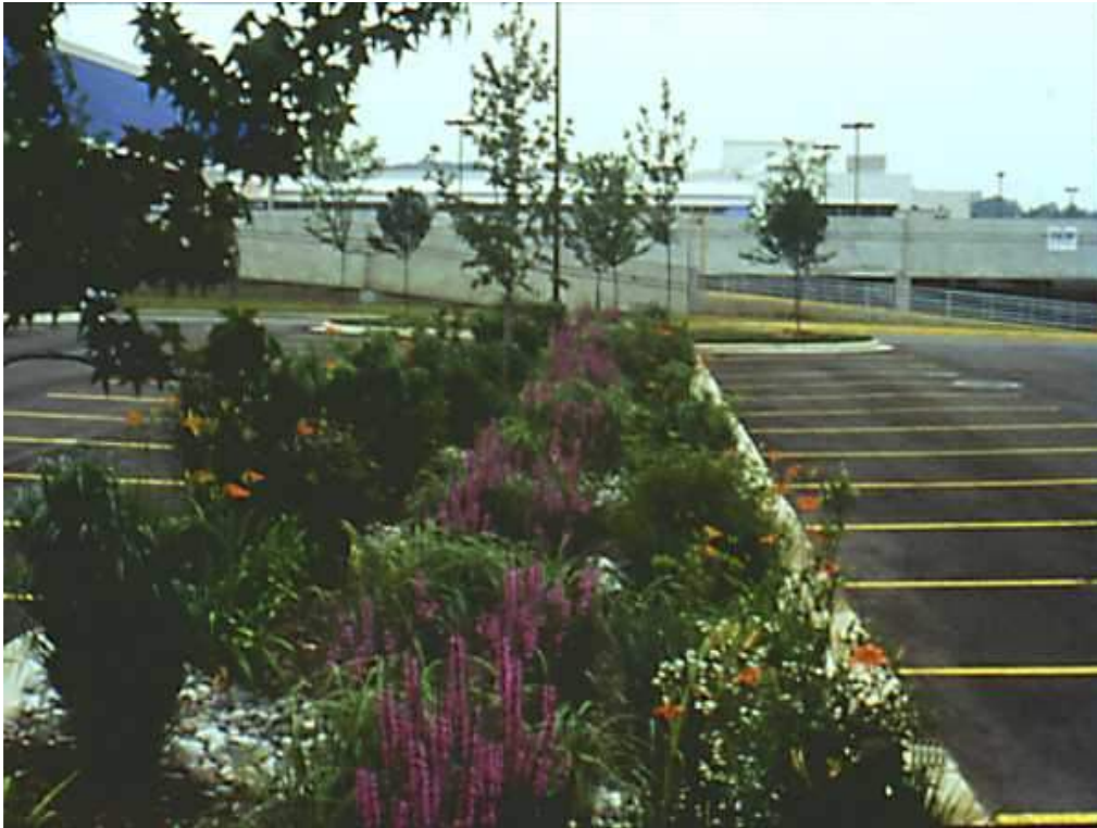
Figure 4-6 Example of Bioretention Landscaping Parking Lot
