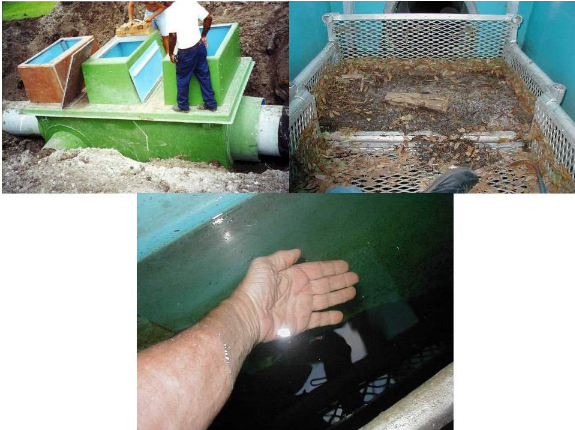
Figure 4-7 Example Second Generation Baffle Box from Suntree Technologies
