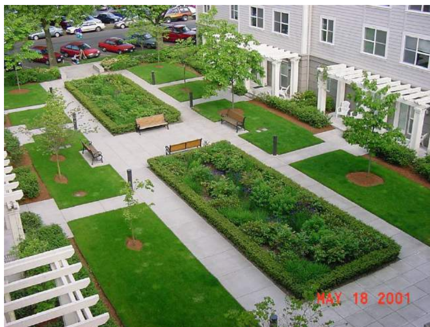
Figure 4-5 Buckman Heights Courtyard with Infiltration Green
