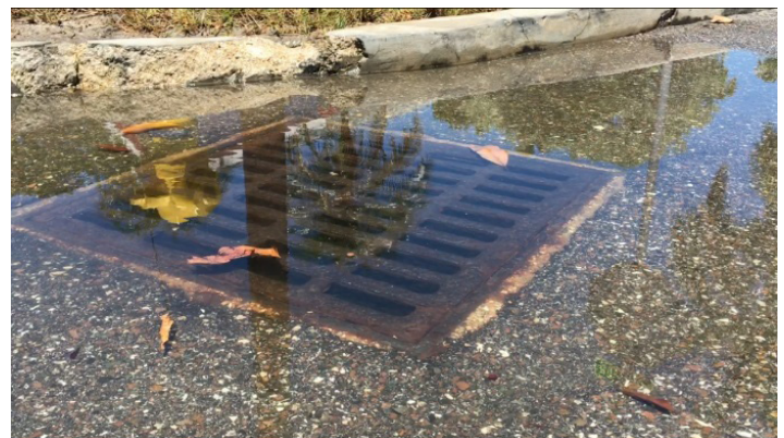
Figure 7. Seawater coming up through a storm drain on Longboat Key during a May 2017 King Tide. Photo credit: SBEP.
