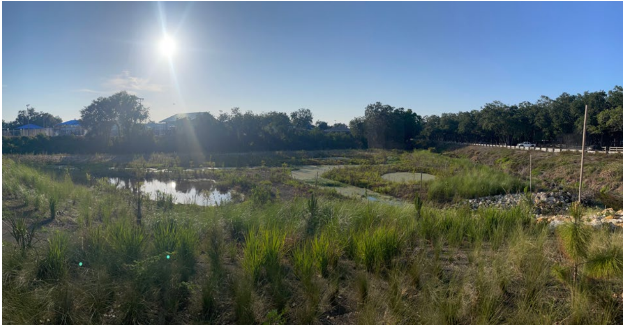
Figure B6 – Stream restoration of Cedar Hammock Creek at GT Bray Park
