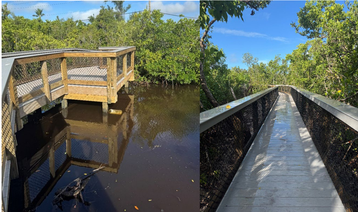
Figure B10 – Completed Boardwalk
