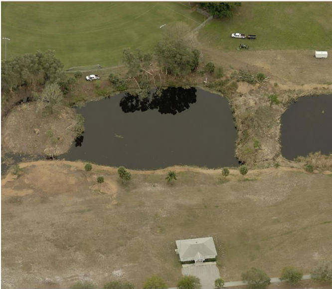
Figure 18 – Aerial view of the stormwater pond to be retrofitted and revitalized at GT Bray Park
