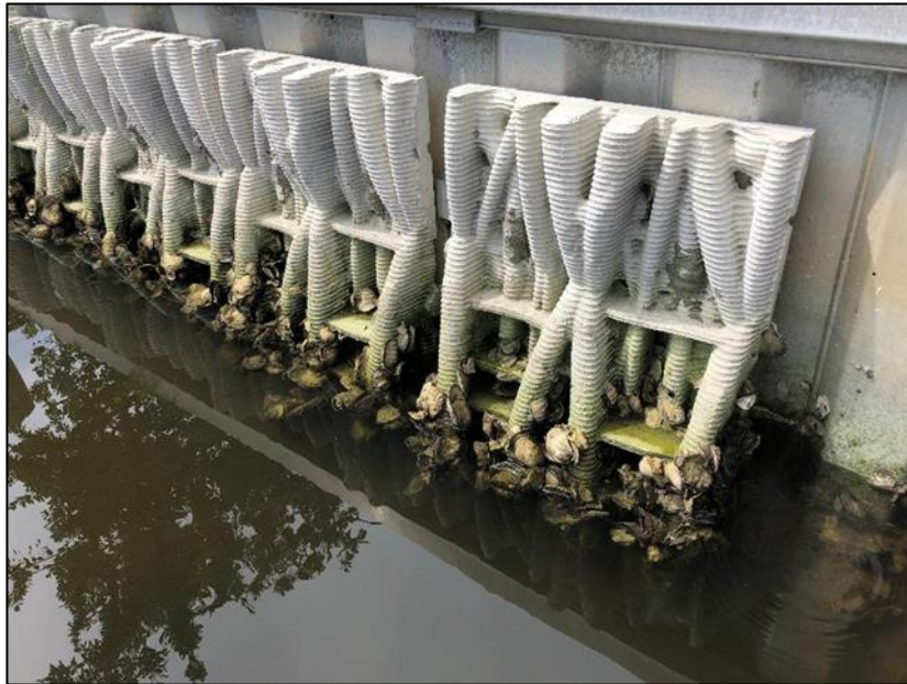
Figure 5 – Photo of a concrete “mangrove panel” attached to the outside of an existing seawall. These mangrove panels would be installed on the recently completed fiberglass seawall at the park.
