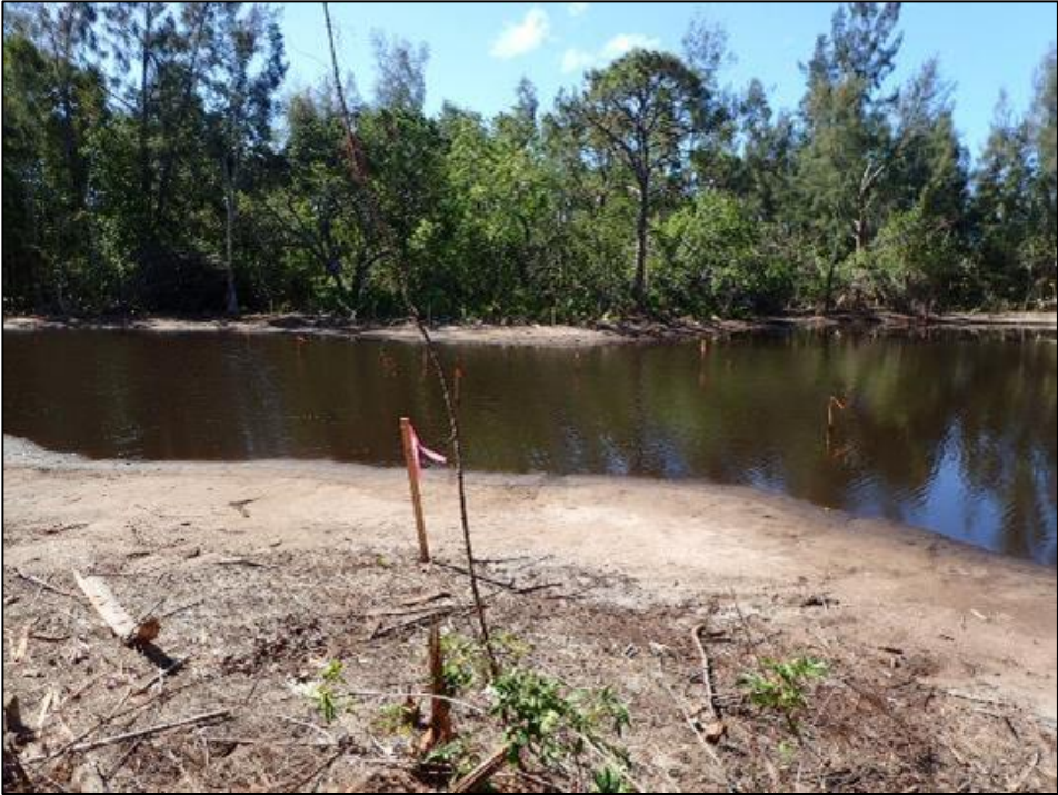
Figure 15 – Land grading at FISH Preserve Phase IV restoration project
