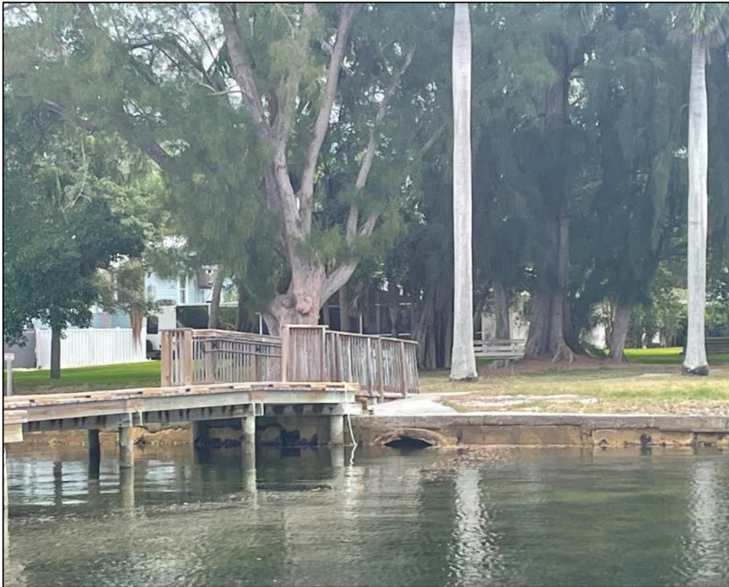
Figure 10 – Overall site plan and potential benefits of proposed Rose Park shoreline restoration project
