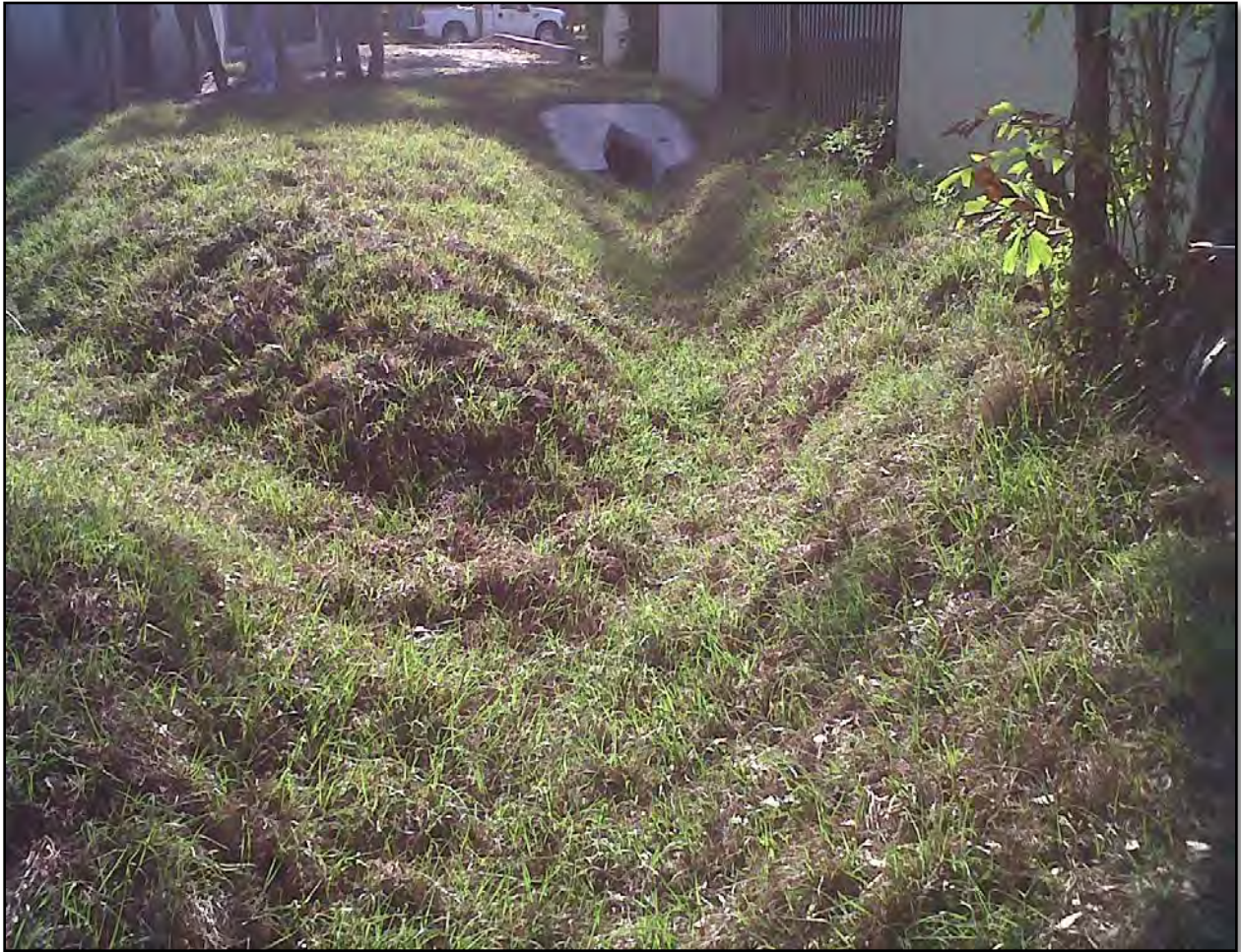
Photograph 16. Original design looking north on the east side of the property where two swales intersected.
