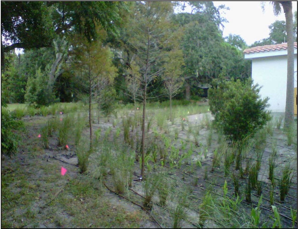
Photograph 22. Planting of the bio-swale including the temporary irrigation system to establish plants.
