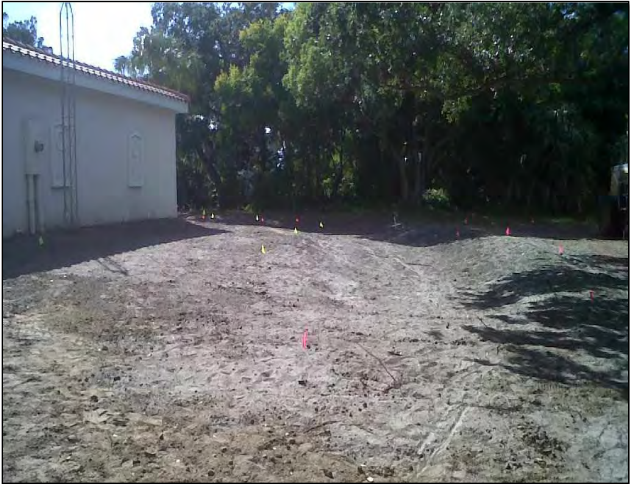
Photograph 25. Area re-graded to stabilize side slopes; maximize bio-swale area; and improve access to lift station.
