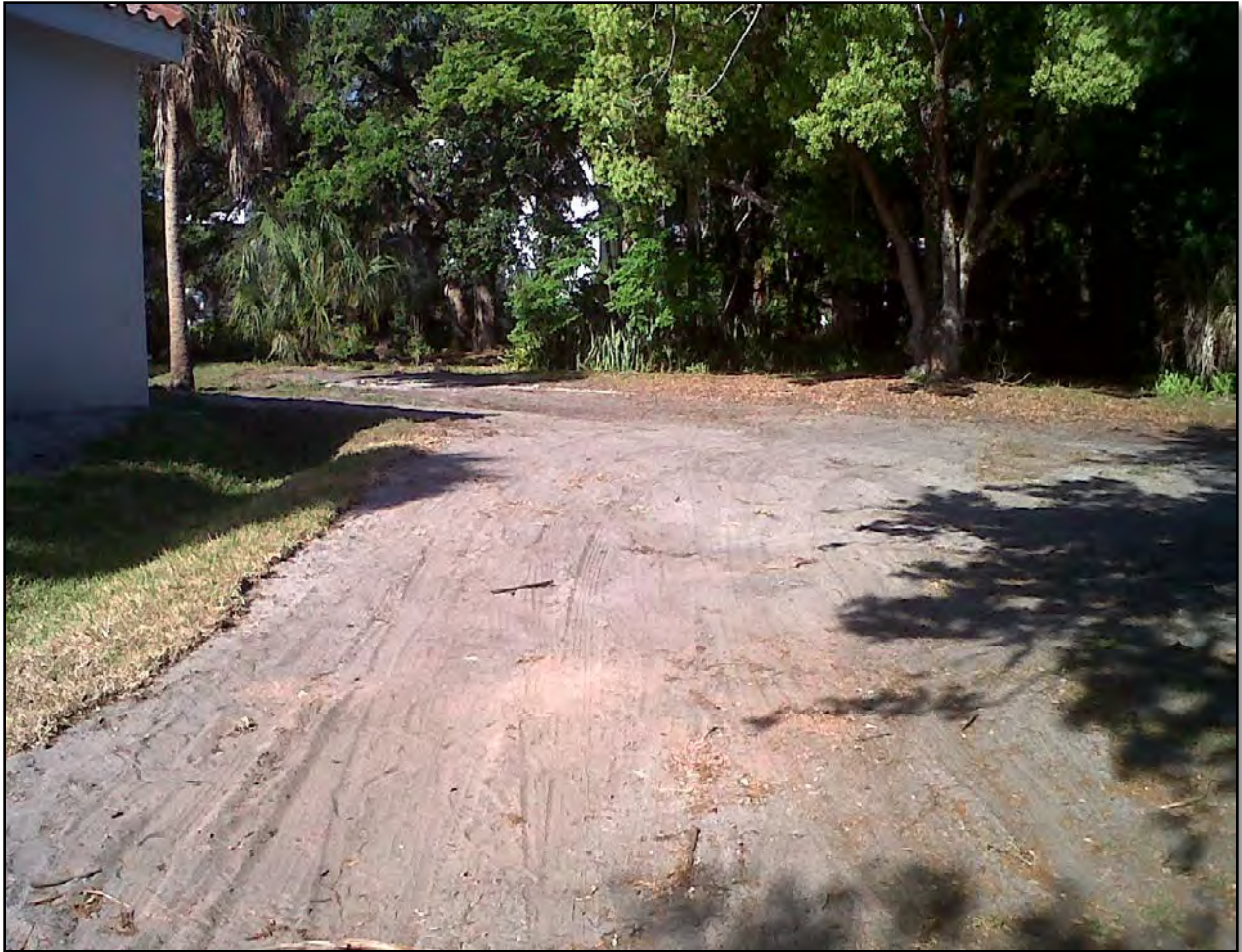
Photograph 24. Original design looking southeast with swale adjacent to structure.
