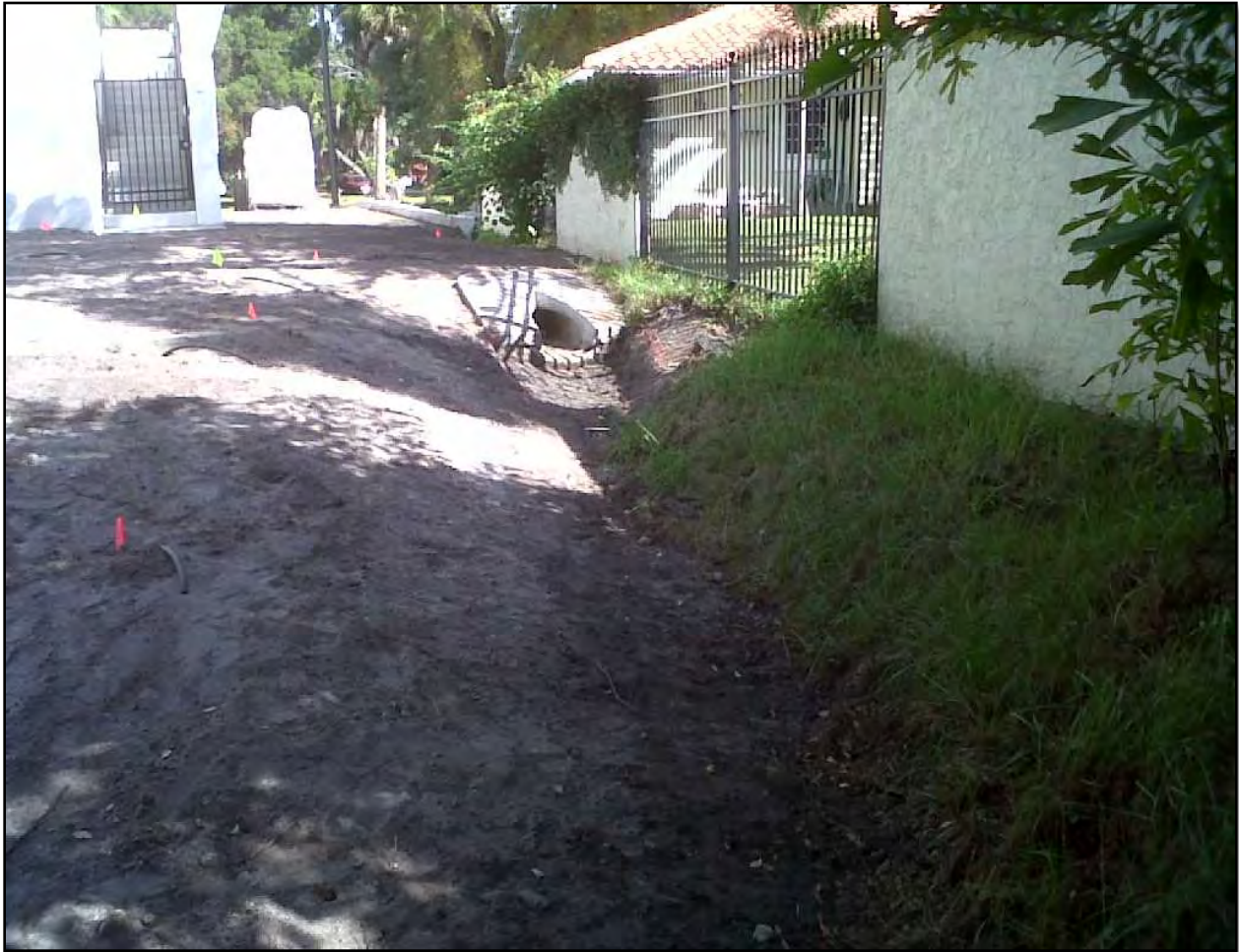
Photograph 17. Area re-graded to remove earthen berm between two swales and increase bio-swale area.
