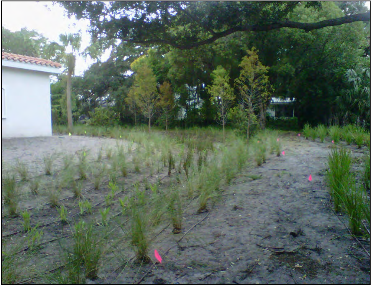
Photograph 26. Planting of the bio-swale including the temporary irrigation system to establish plants.
