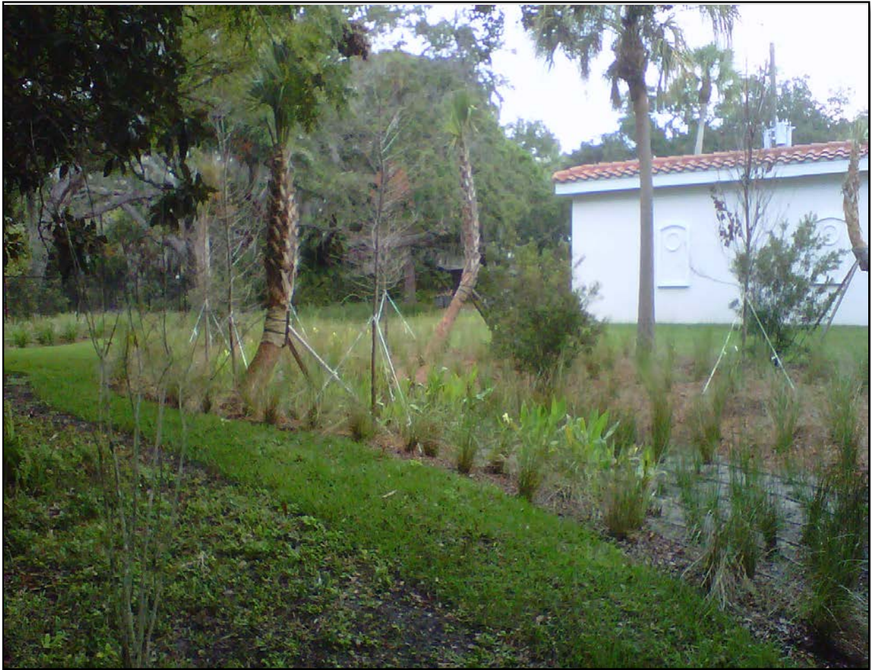
Photograph 23. Completed bio-swale three months after construction.
