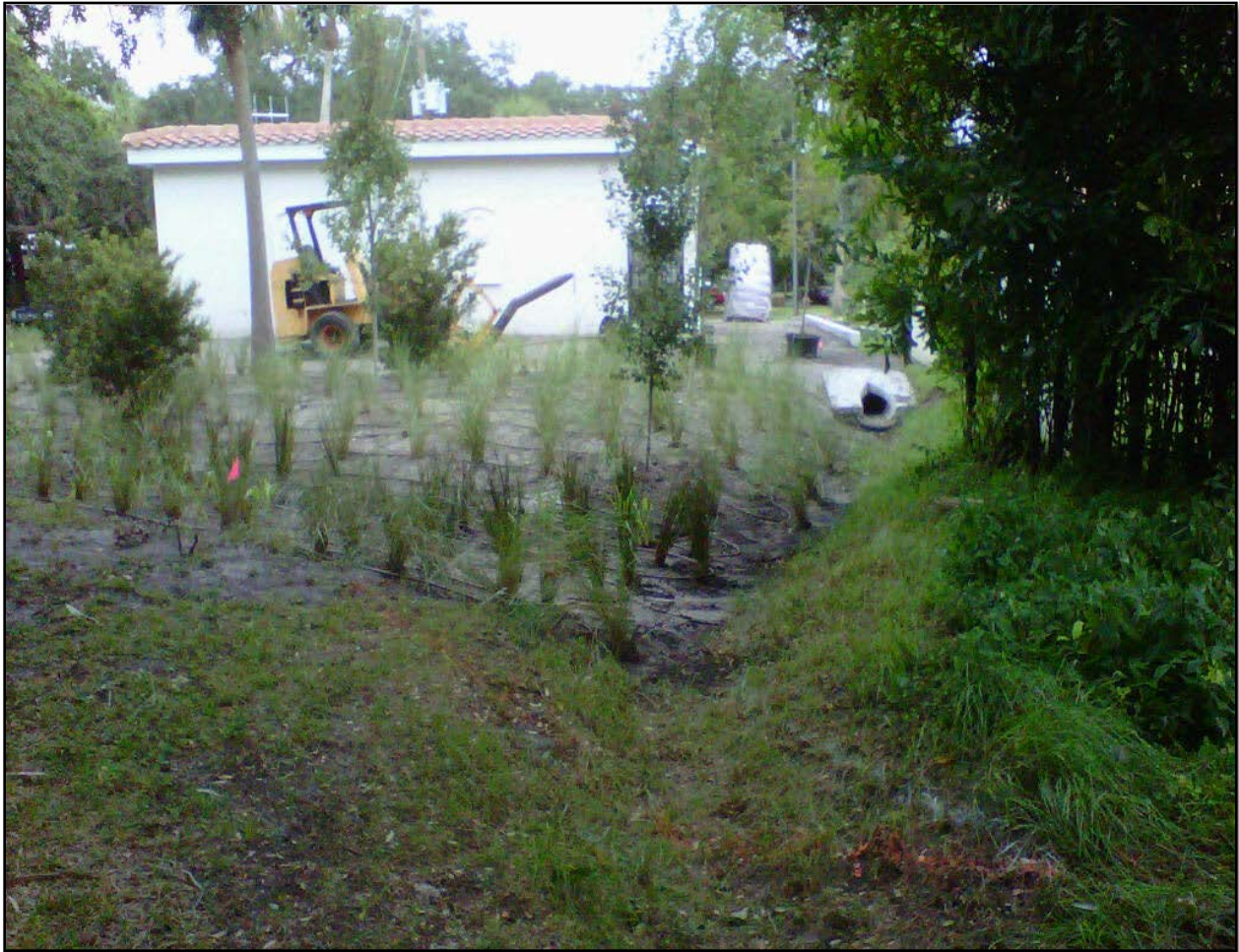
Photograph 18. Planting of the bio-swale including temporary irrigation system for establishing plants.
