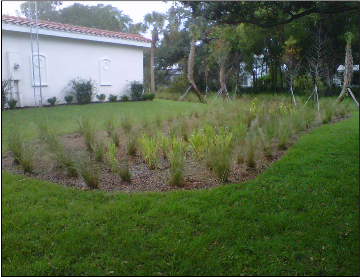
Photograph 27. Completed bio-swale three months after construction.
