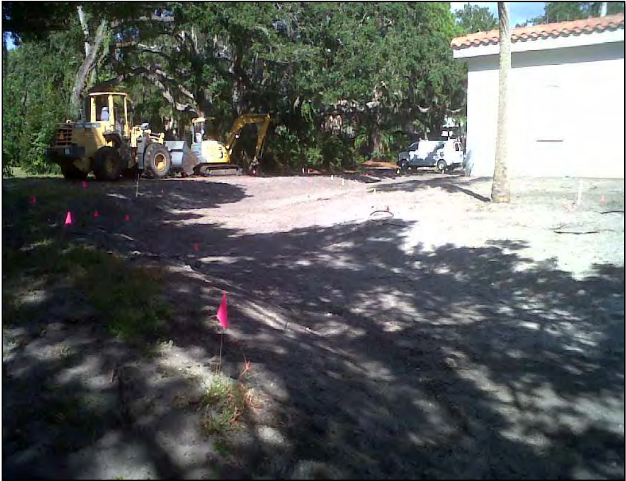
Photograph 21. Area re-graded to stabilize side slopes; maximize bio-swale area; and improve access to lift station.
