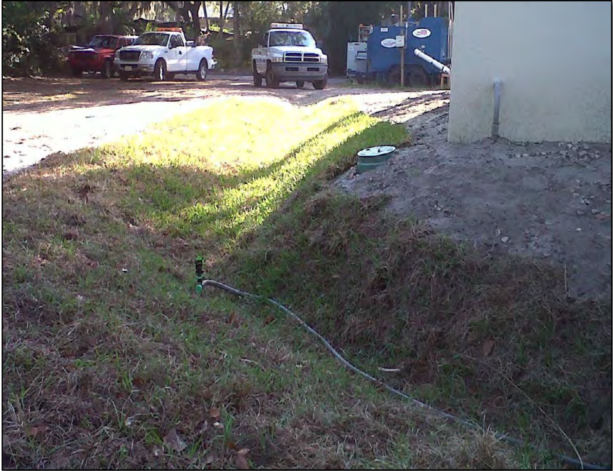
Photograph 20. Original design looking northwest at main swale adjacent to structure.
