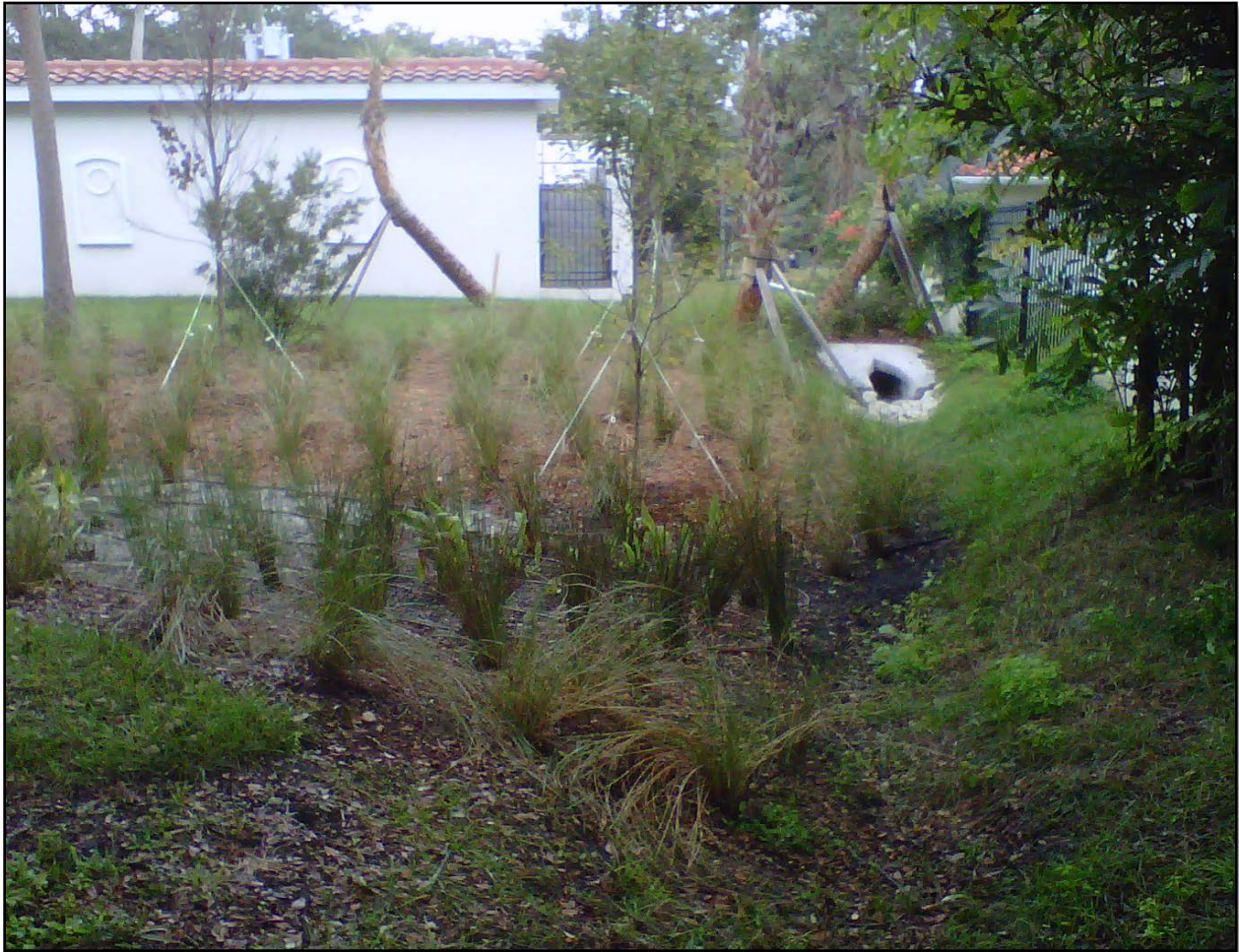
Photograph 19. Completed bio-swale two months after construction.
