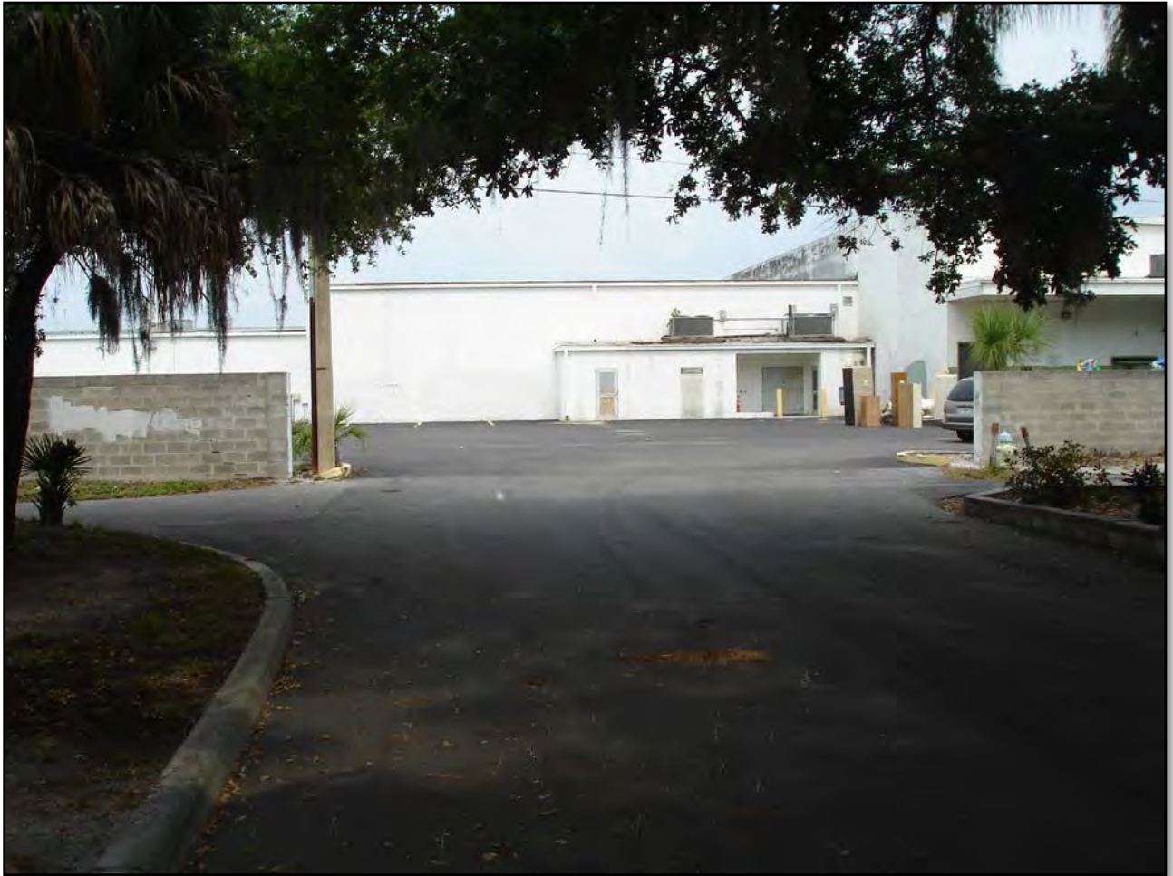
Photograph 11. Site 6 existing conditions looking east.
