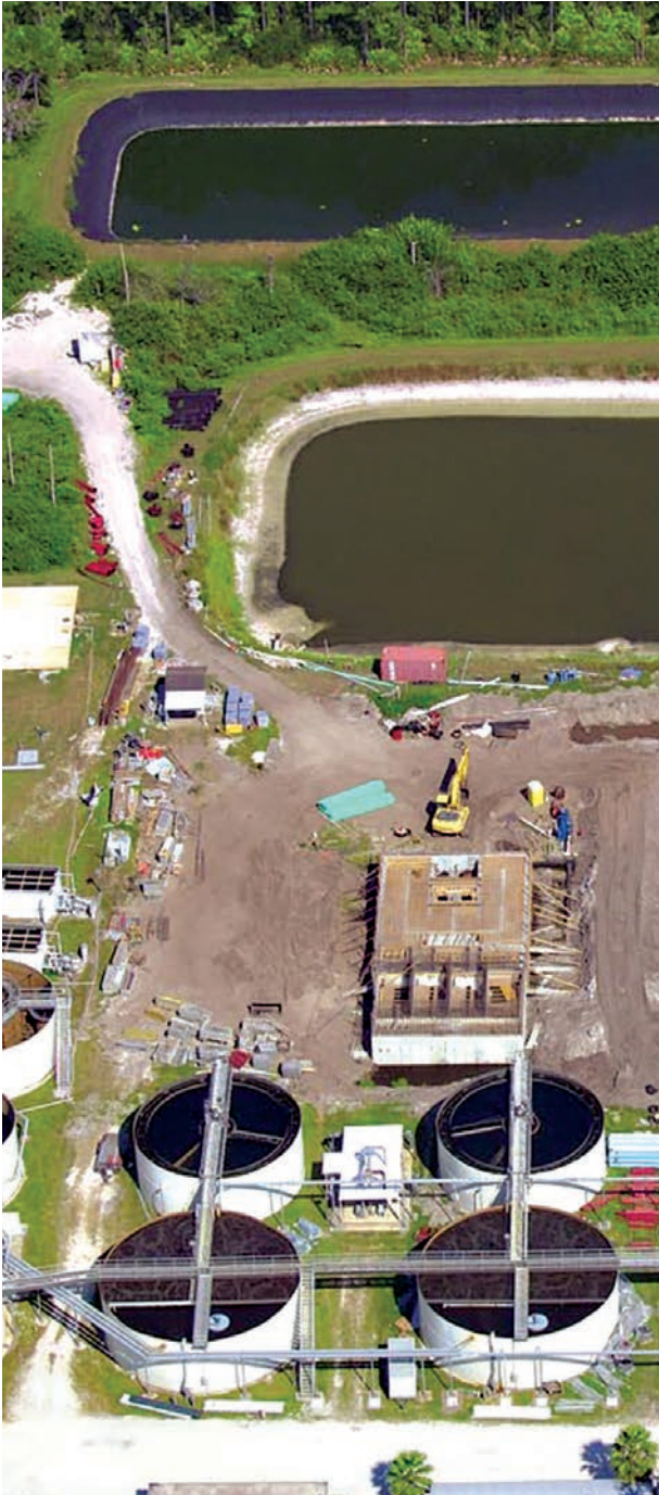
Fruitville Water Reclamation Facility. (Sarasota County)
