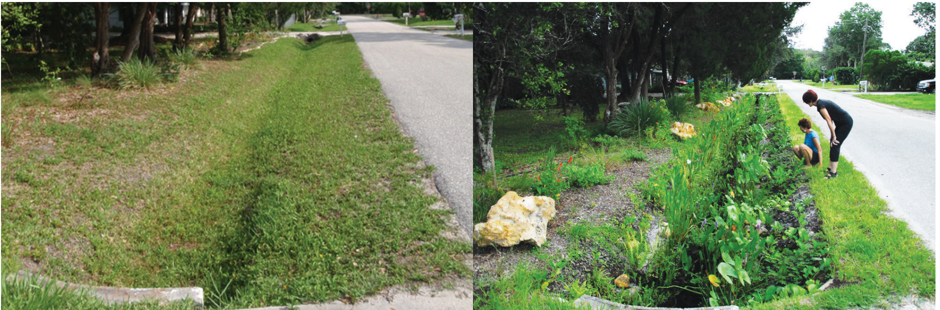
Example of grassy swale (left) and same swale with native plants (right) to increase evaporation of water and increase pollutant removal. (SBEP)
