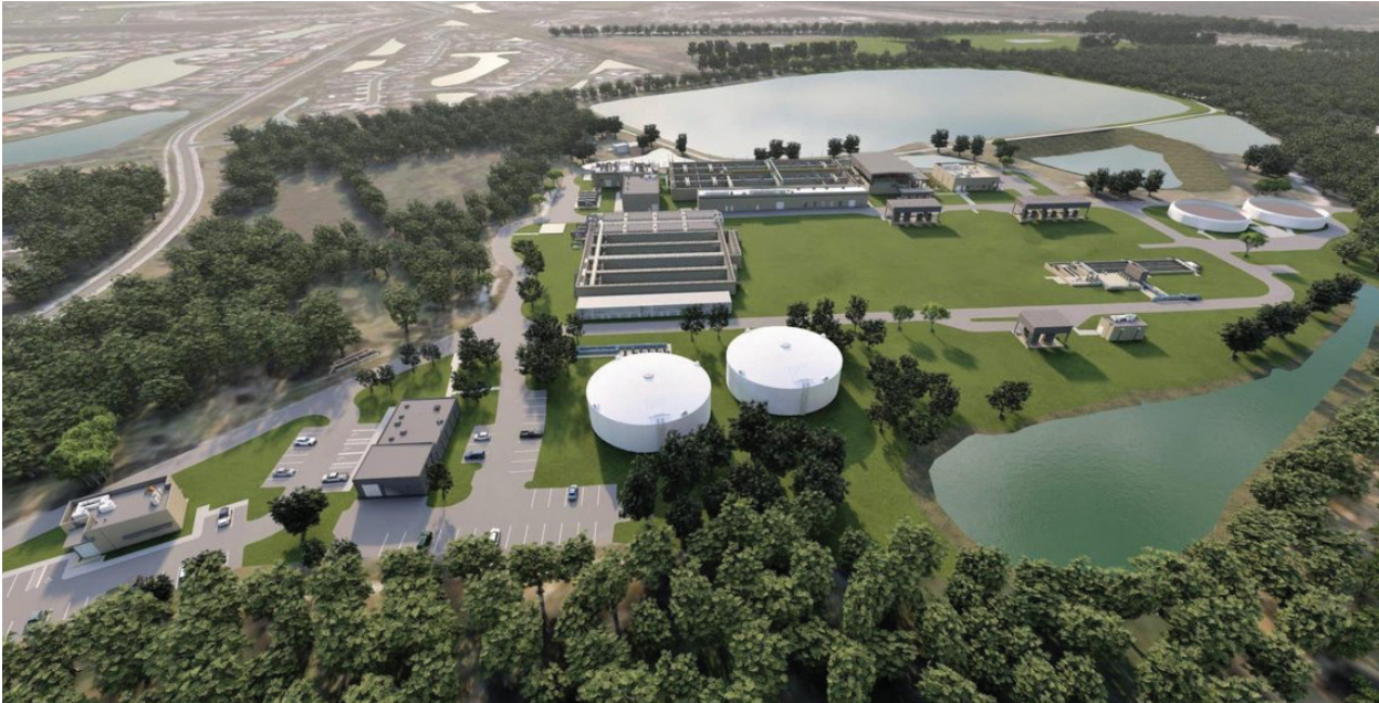
Bee Ridge Water Reclamation Facility, Sarasota County. (Sarasota County)
